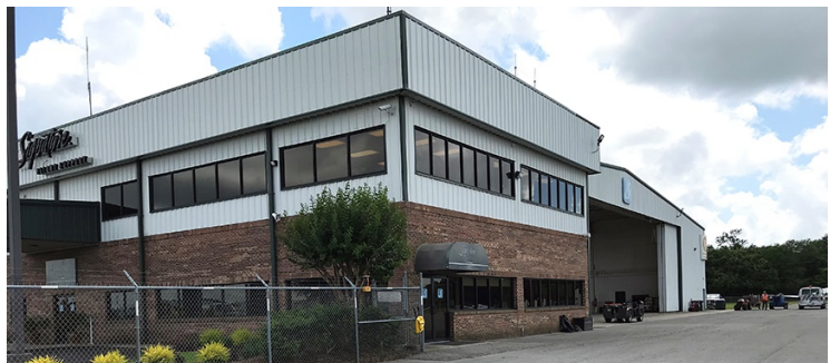
Figure 9.2: Signature FBO Building
